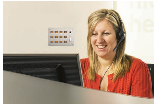
A reception desk equipped to handle emergency communications with people in disabled refuges
